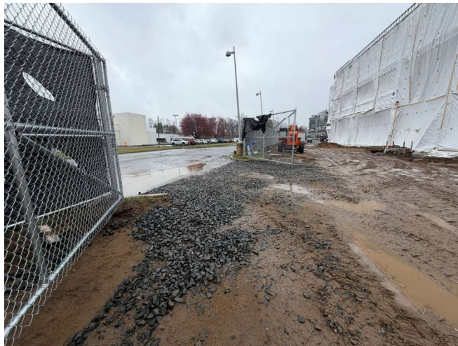
Pictures 3: Construction Entrance (N)
