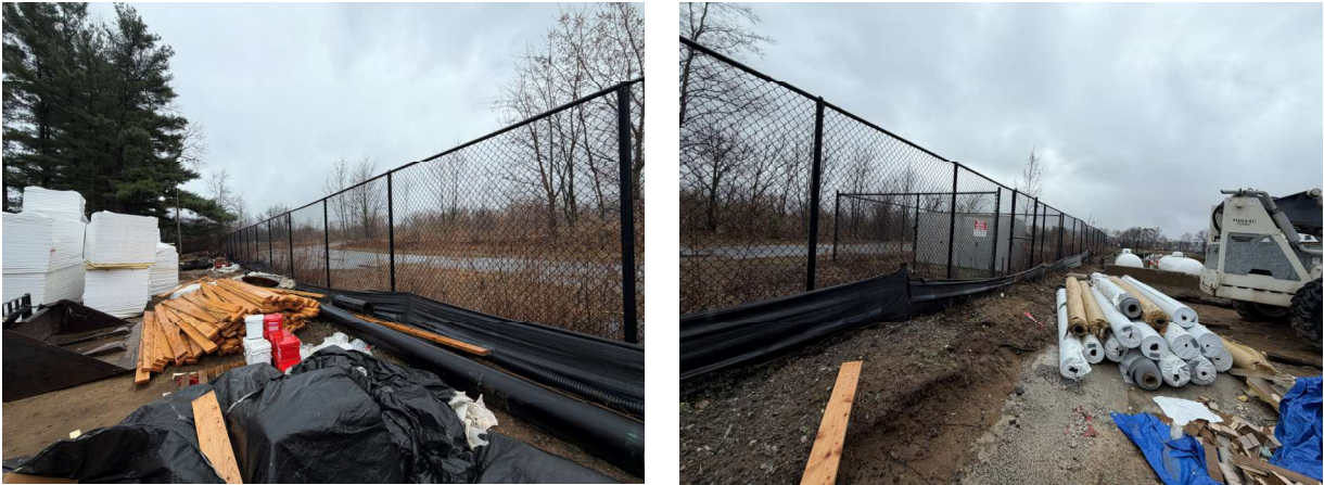
Pictures 4-5: Silt Fence (W)
