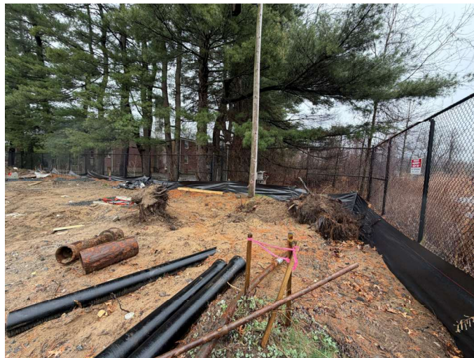
Picture 6: Silt Fence (S)
