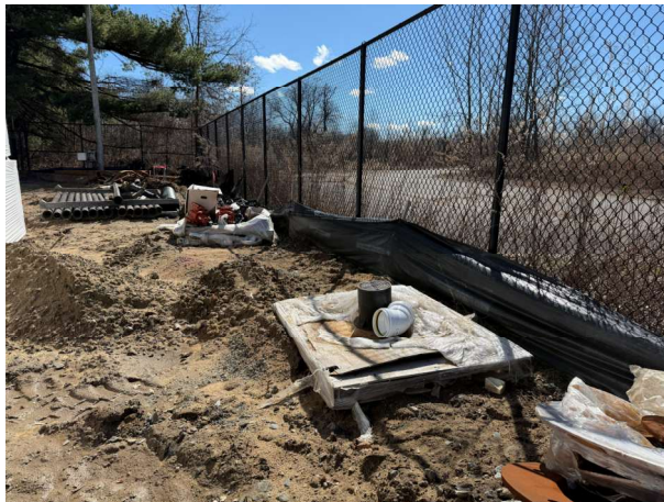
Picture 5: Silt Fence (W) – Repair Silt Fence
