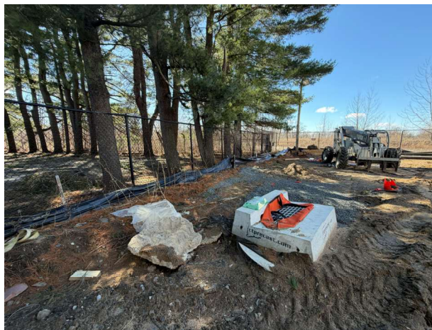
Picture 6: Silt Fence (S) – Restaple Sections to Posts
