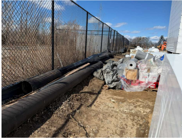
Picture 4: Silt Fence
