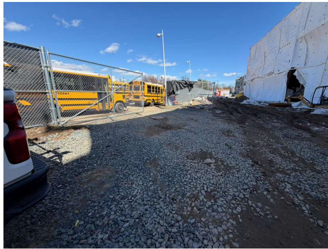
Picture 3: Construction Entrance (N)
