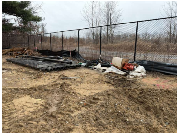
Picture 5: Silt Fence (W) – Restaple Sections to Posts
