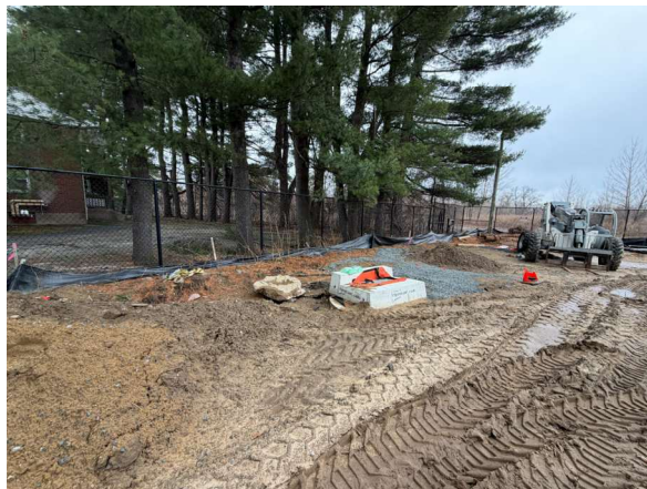
Picture 6: Silt Fence (S) – Restaple Sections to Posts
