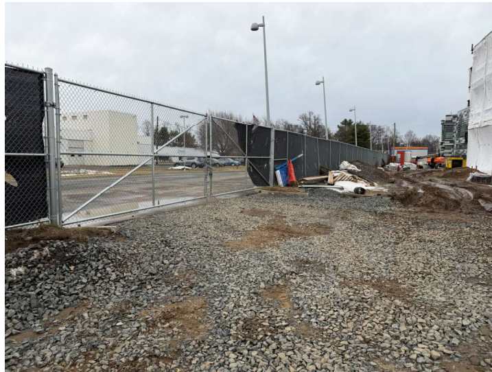
Picture 1-3: Construction Entrances
