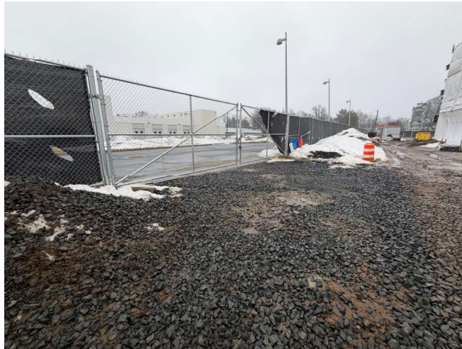
Picture 1-3: Construction Entrances
