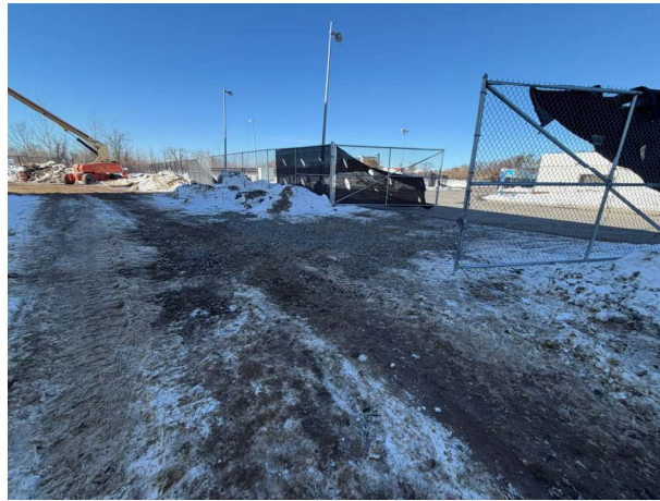
Picture 1-3: Construction Entrances
