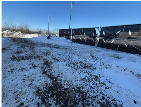
Picture 1-3: Construction Entrances
