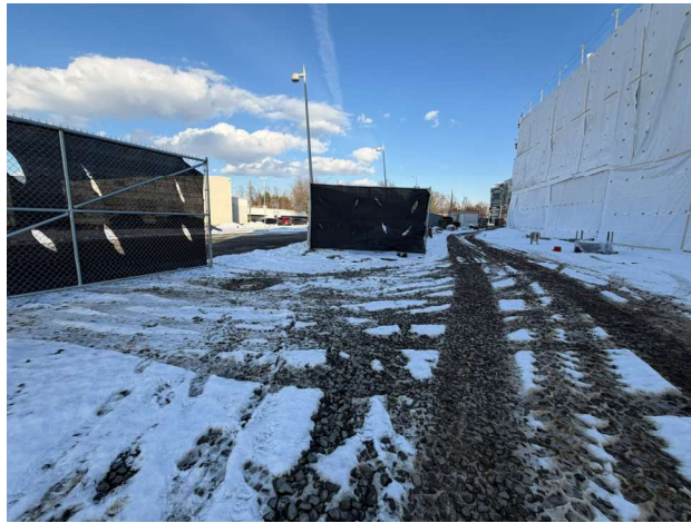
Picture 1 -3: Construction Entrances
