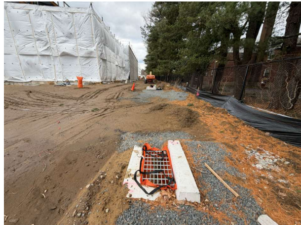
Pictures 2-3: Installation of Catch Basins
