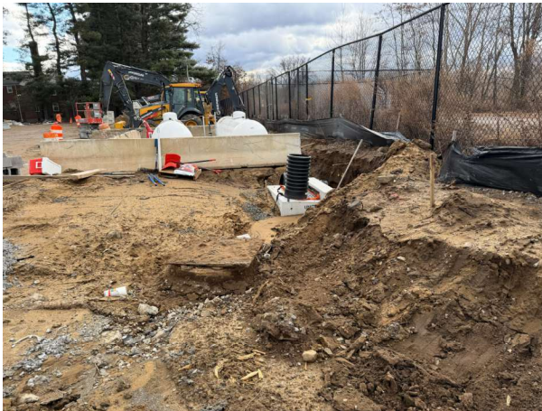
Pictures 2-3: Installation of Catch Basins
