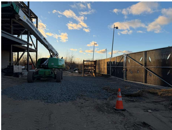
Picture 3: North Gate - Construction Entrance
