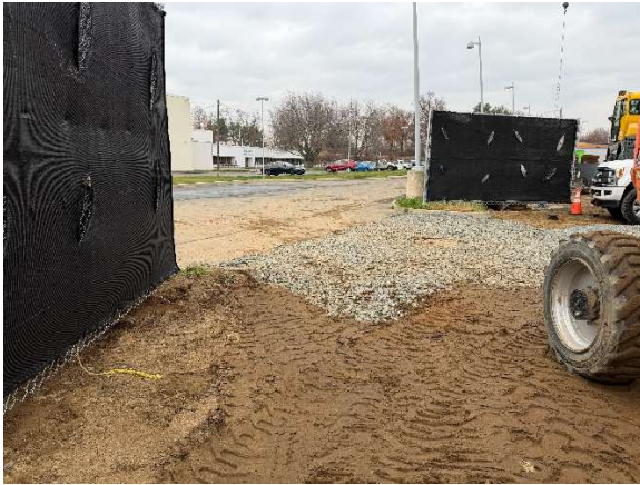
Pictures 4 & 5: North Gate - Construction Entrance Pad
