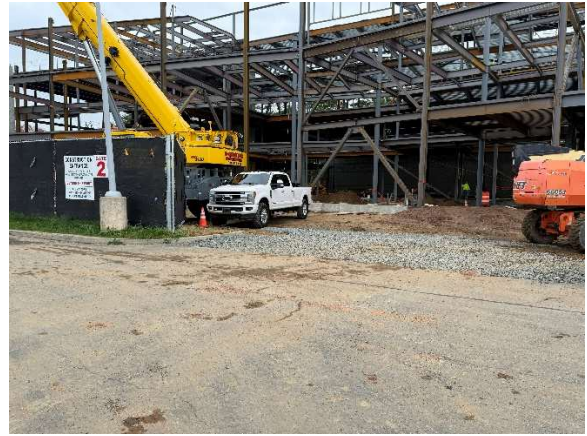
Pictures 4 & 5: North Gate - Construction Entrance Pad
