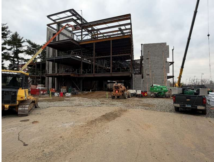
Picture 1: Main Gate - Construction Entrance Pad
