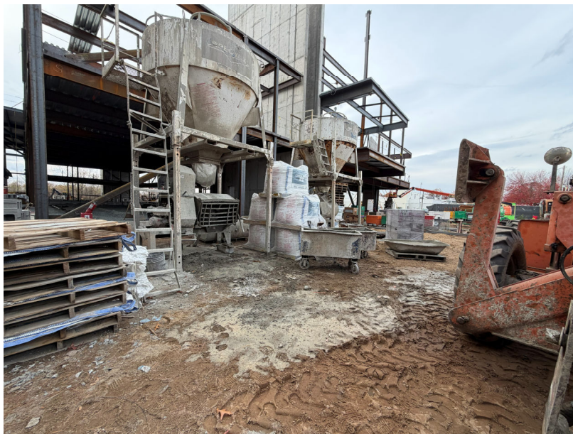
Picture 2: Concrete Activities
