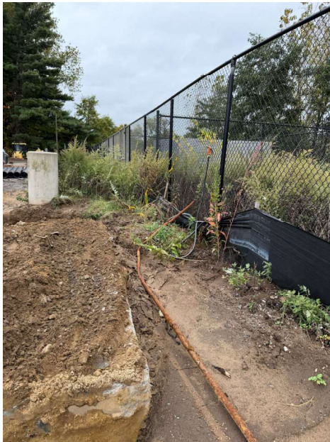
Pictures 2 & 3: Silt Fence - Along Western Fence Line
