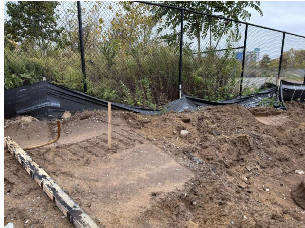
Pictures 2 & 3: Silt Fence - Along Western Fence Line
