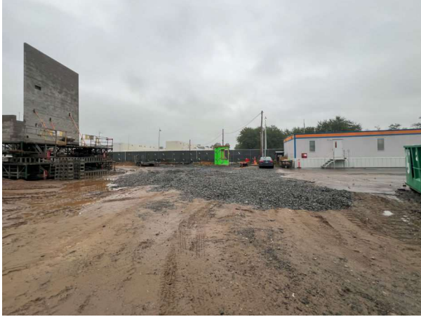
Pictures 1 & 2: Construction Entrance Pad Extended
