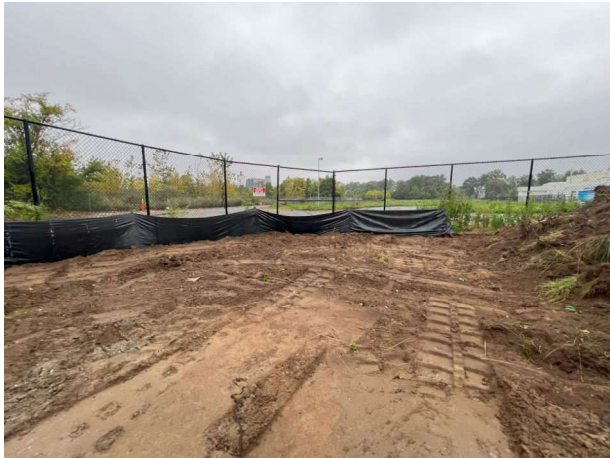
Pictures 3 & 4: Silt Fence - Northwest Corner and Along Western Edge of Site
