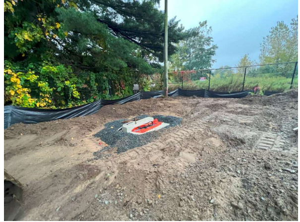
Pictures 5 & 6: Inlet Protection at Catch Basin
