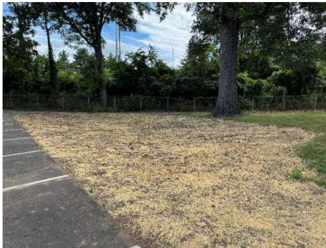
Picture 2: Soil stockpile area has been stabilized.
