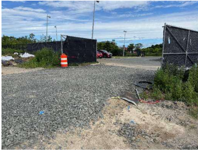
Picture 3: Construction entrance in good condition.
