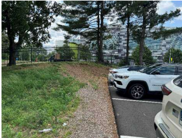
Picture 1: Seed and stabilize or install temporary erosion control measures if left undisturbed for 30 days.
