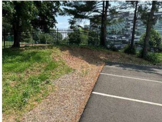
Picture 1: Seed and stabilize or install temporary erosion control measures if left undisturbed for 30 days.
