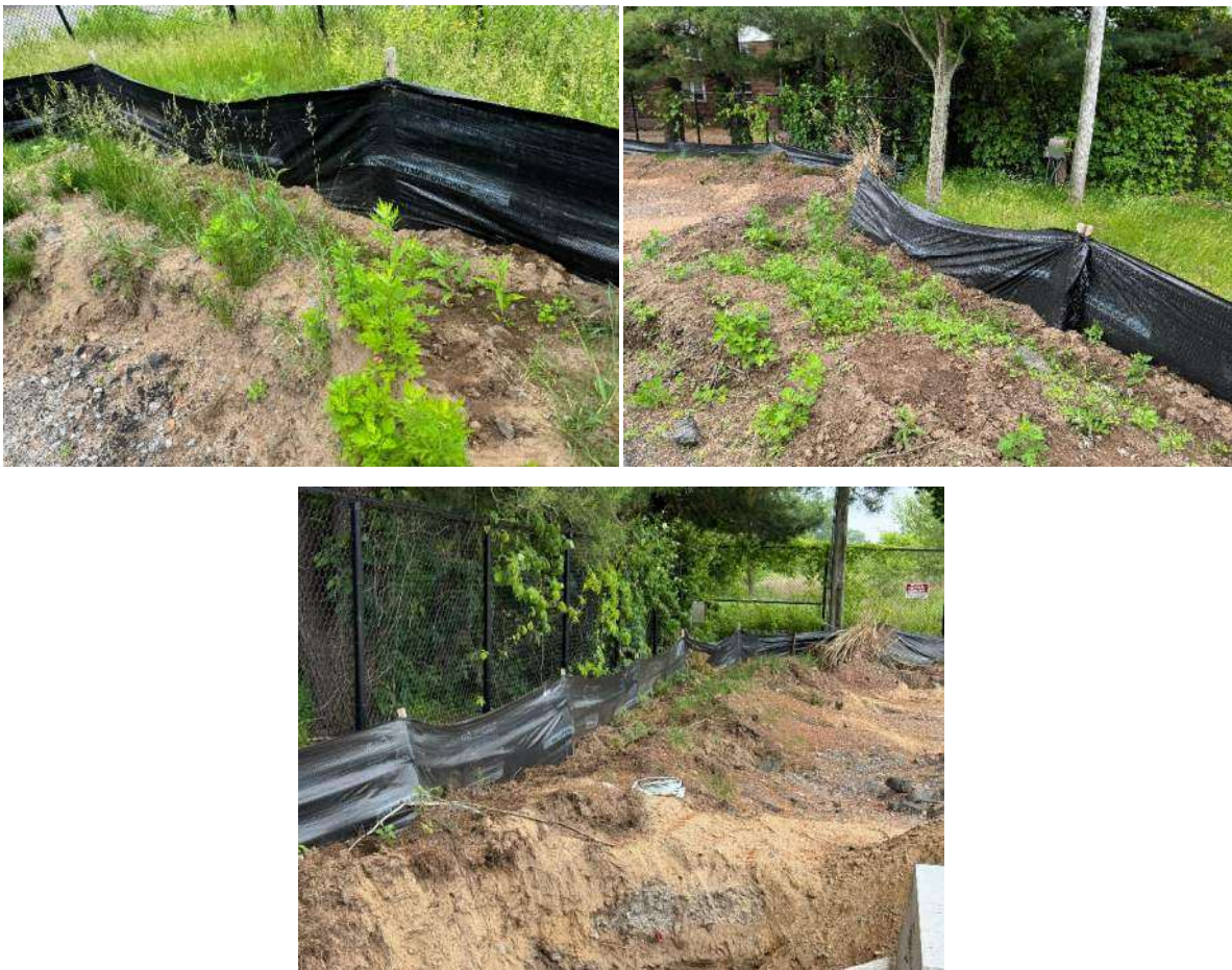
Picture 4, 5 & 6: Silt fence has been fixed throughout the site.
