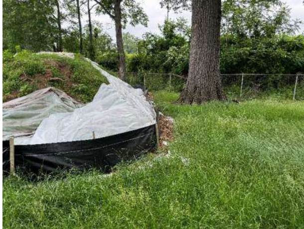
Picture 1: Silt Fence has been fixed around stockpile.
