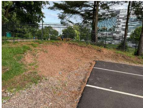
Picture 2: Seed and stabilize or install temporary erosion control measures if left undisturbed for 30 days .
