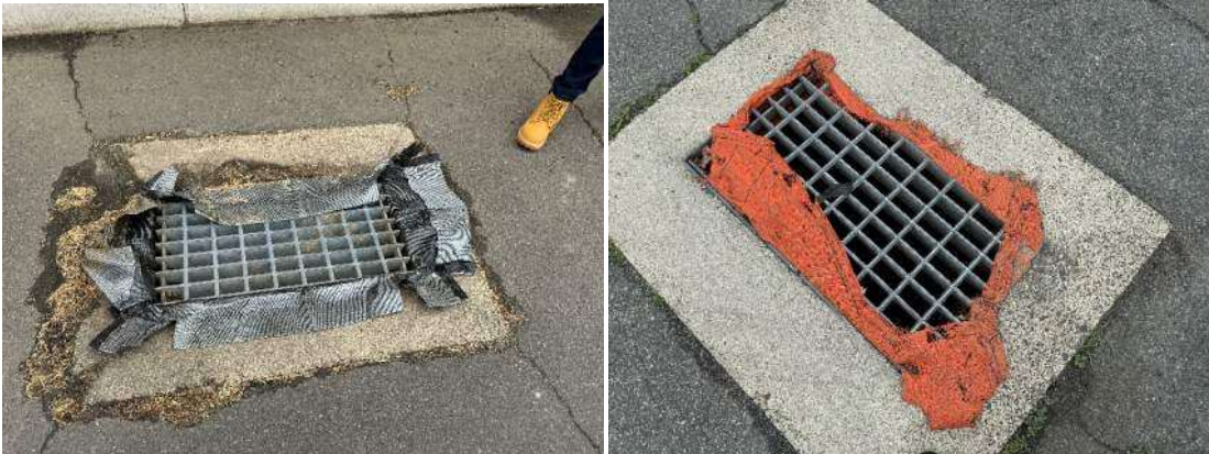
Picture 3 & 4 : Silt sacks have been replaced or cleaned throughout site.
