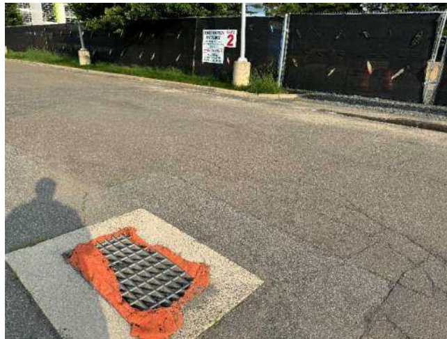
Picture 3, 4 & 5 : Remove debris and standing water in catch basins.
