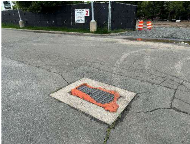
Picture 3, 4 & 5 : Remove debris and standing water in catch basins.
