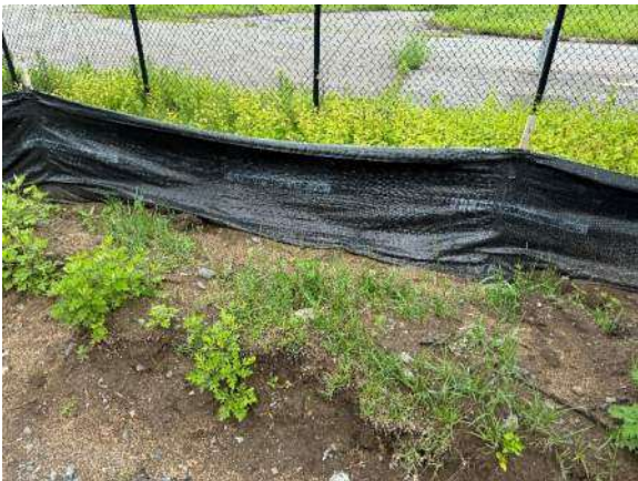
Picture 6 & 7: Silt fence not buried.
