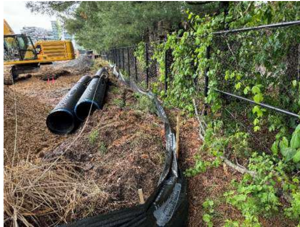
Picture 8: Silt fence needs to be reattached to stake along project edge.
