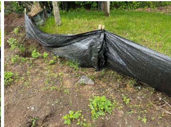
Picture 6 & 7: Silt fence not buried.
