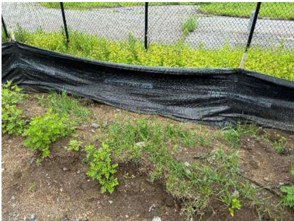
Picture 6 & 7: Silt fence not buried.
