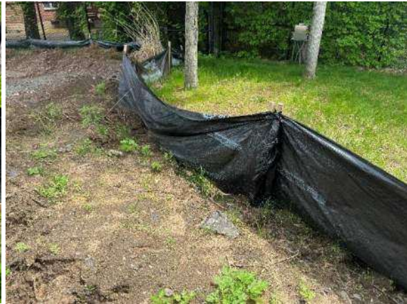
Picture 5: Silt fence not buried.
