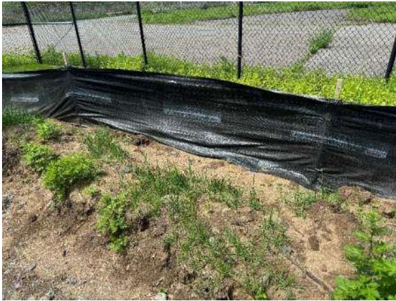
Picture 5: Silt fence not buried.
