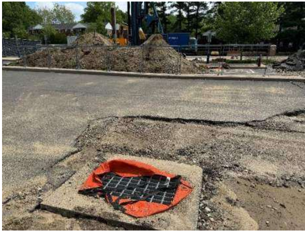
Picture 3 & 4: Remove debris and standing water in catch basins.
