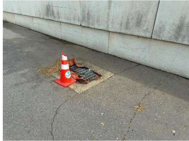
Picture 3 & 4: Remove debris and standing water in catch basins.
