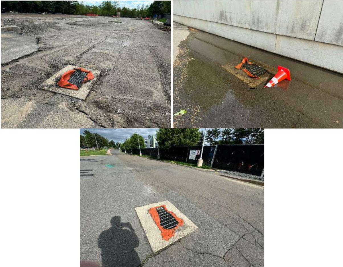
Picture 3 & 4: Remove debris and standing water in catch basins.
