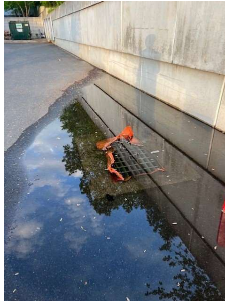
Picture 1 & 2: Remove debris and standing water in catch basins.
