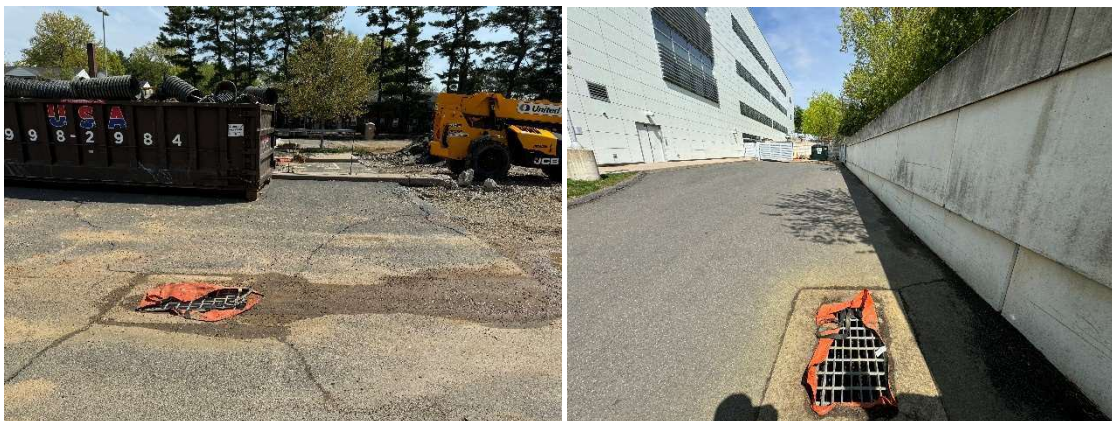
Picture 3 & 4: Remove debris and standing water in catch basins.
